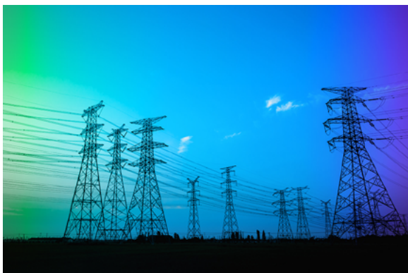
ELECTRICAL GRID INSTALLATIONS
