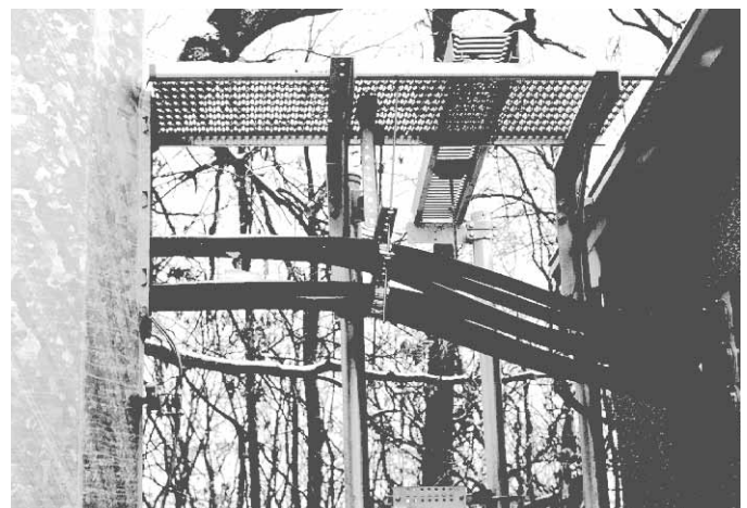
Cable run from monopole to equipment building
