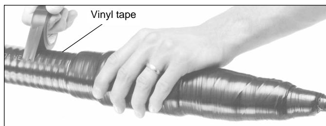
Standard Connector/Splice Weatherproofing Kit
